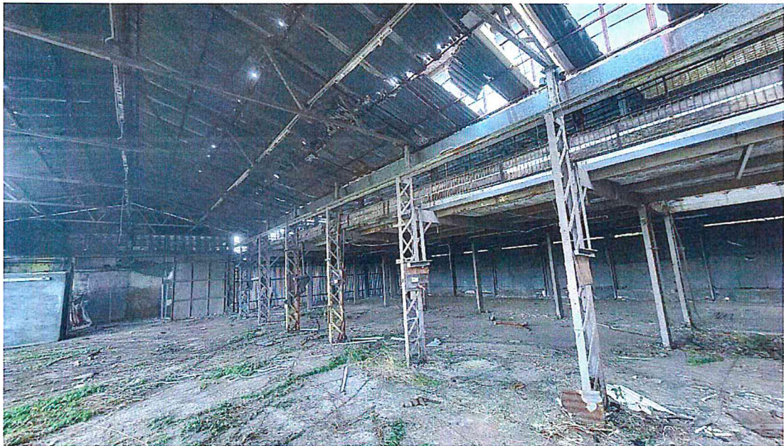
Internal View of an Existing Structure
