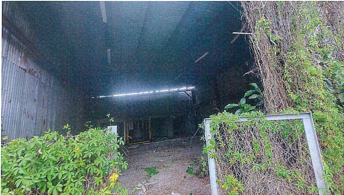
Internal View of an Existing Structure
